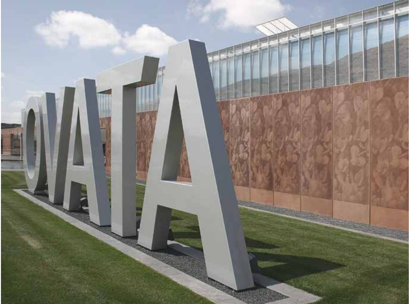
OVATA BUILDING RECKLI PHOTO-ENGRAVING BLEISWIJK NETHERLANDS, 2007 IMMEUBLE OVATA RECKLI PHOTOGRAVURE BLEISWIJK PAYS-BAS, 2007
