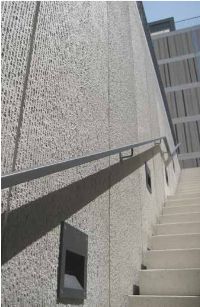
RESIDENTIAL BUILDING RECKLI STANDARD 2/108B INDUS LAUSANNE SWISS, 2011 ENSEMBLE DE LOGEMENTS RECKLI STANDARD 2/108B INDUS LAUSANNE SUISSE, 2011
