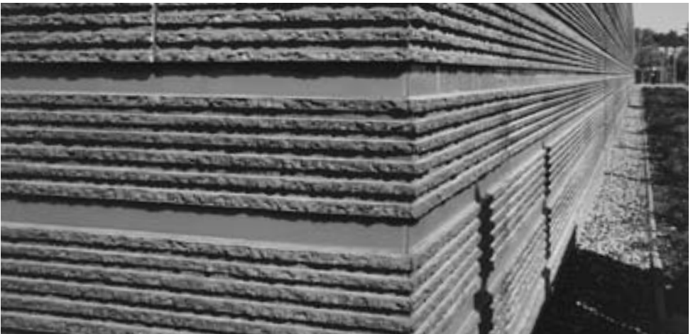
COVE WITH CHAMFER, MIDDLE IN CONCRETE
