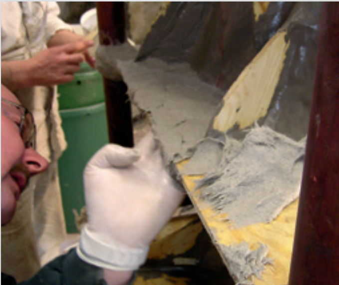
19 | Applying the reinforcement using EP-F Type VB supporting material
