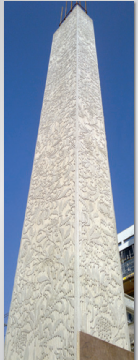
Tendrilled ornament – CNC milling technology with PUR elastomer moulds – white concrete elements
