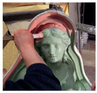
17 Applying the third silicone layer to the second half of the mould
