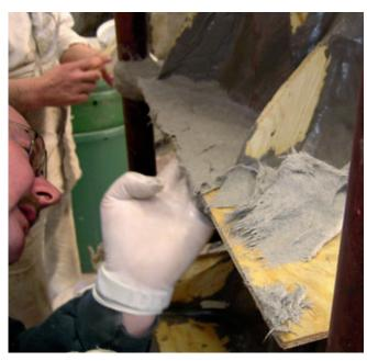
19 Applying the reinforcement using EP-F Type VB supporting material
