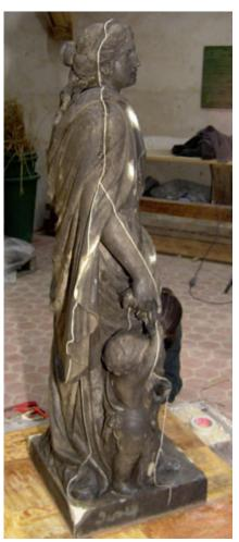
2 Paste applied as a rib to the parting lines
