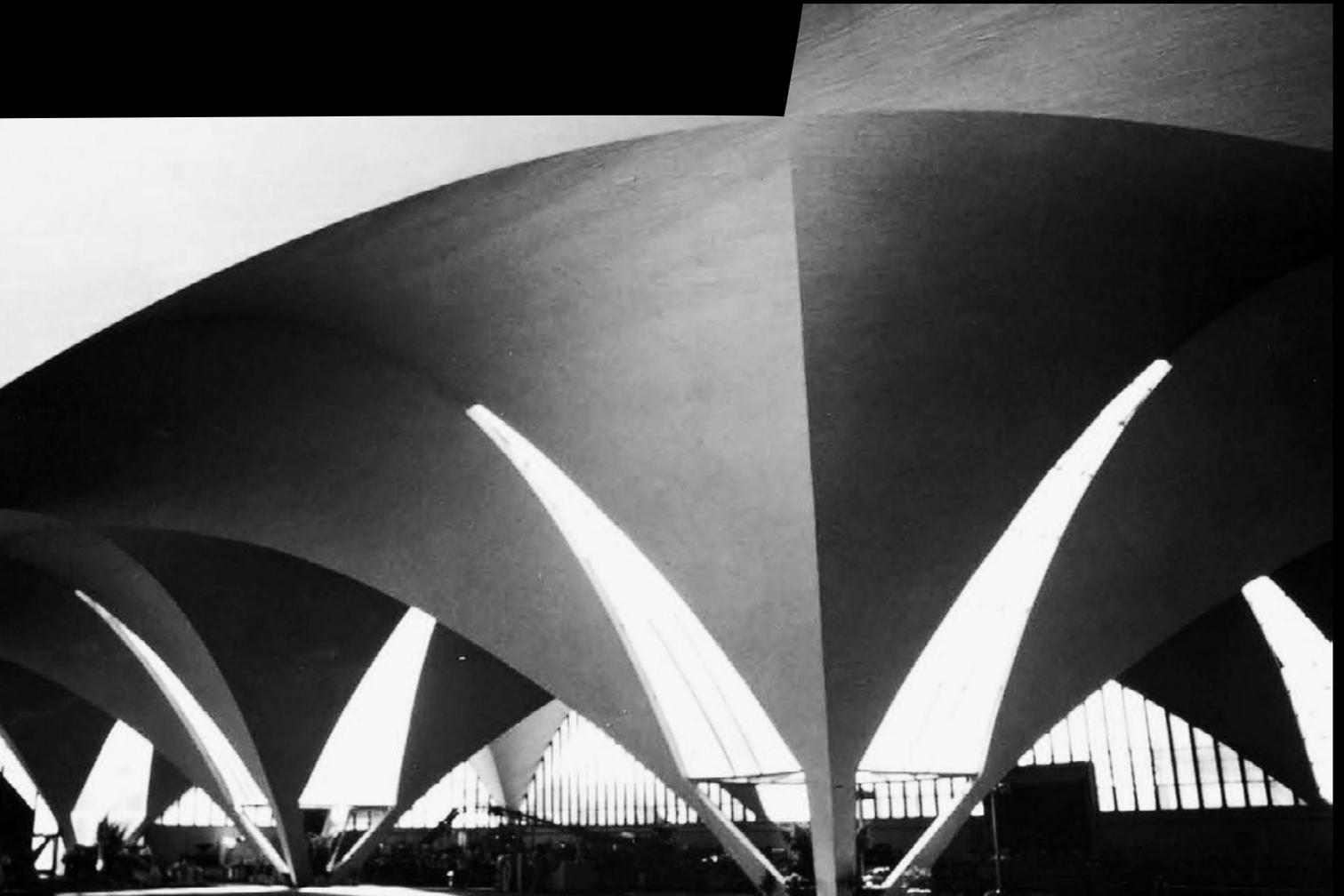
Félix Candela was an architect, but his real passion was engineering. He perfected the hyperbolic paraboloid (hypar) roof, and used it to create groundbreaking buildings of breathtaking lightness and elegance.
