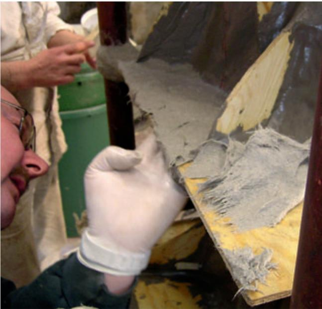
19 Applying the reinforcement using EP-F Type VB supporting material
