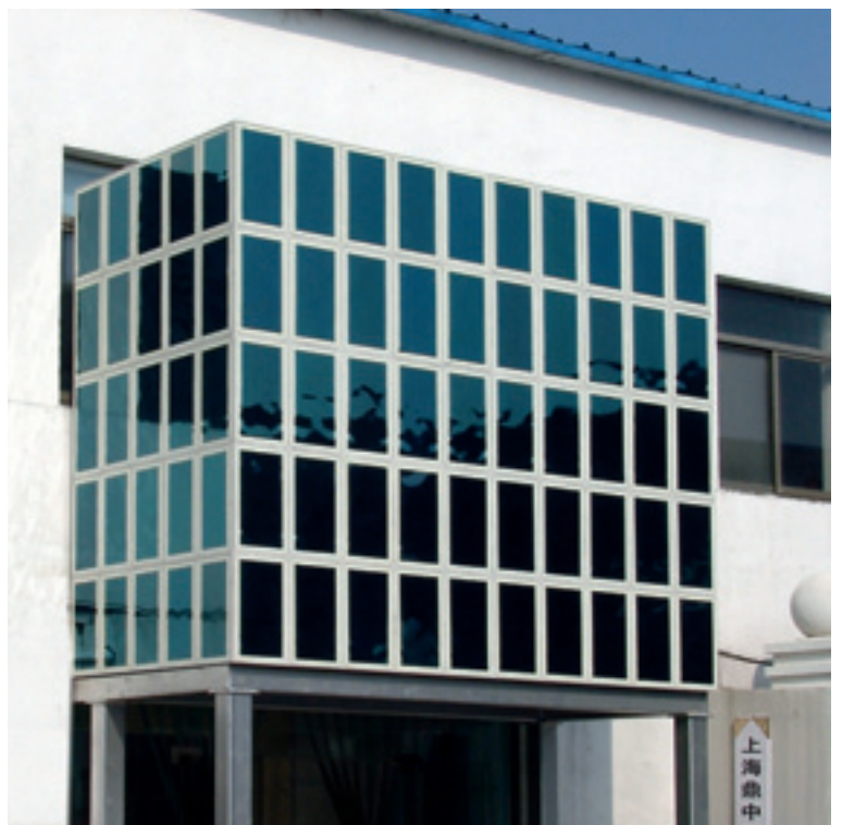
Test installation in Shanghai/China
